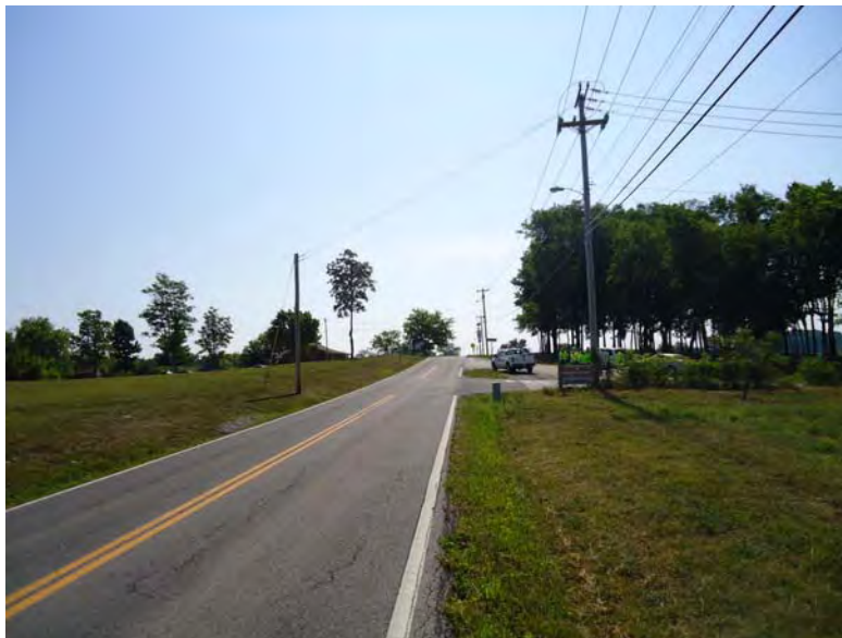
6/22/12: Looking east on State Route 247 towards the intersection of State Route 247 and Cleburne Road. (L.M. 17.20).
